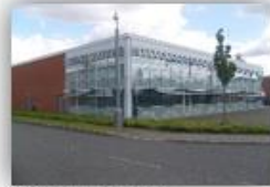
런던 Cell Processing Center
